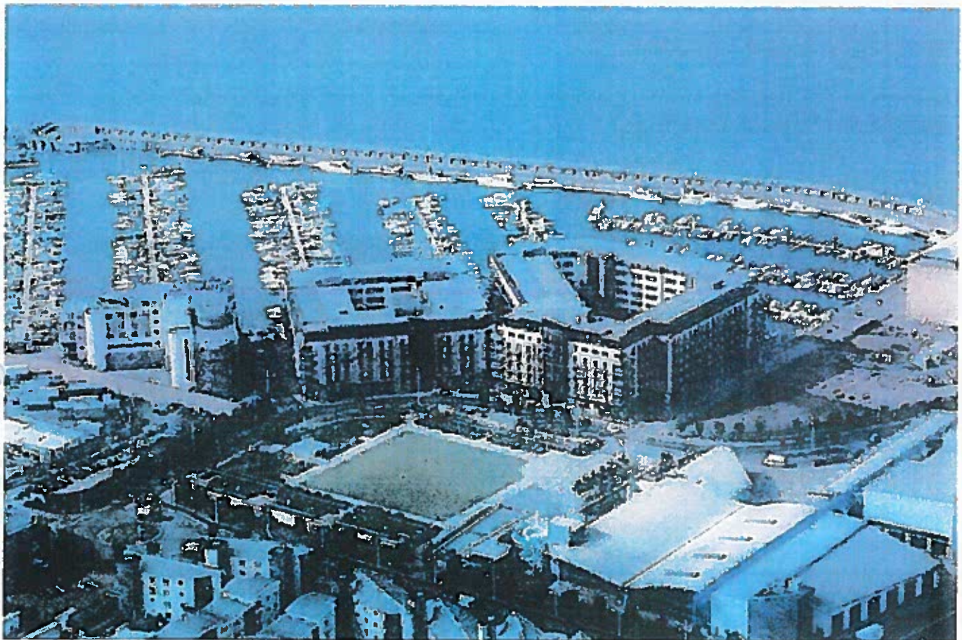
The area of land sold by Le Pas Holdings was developed into the Castle Quay complex
